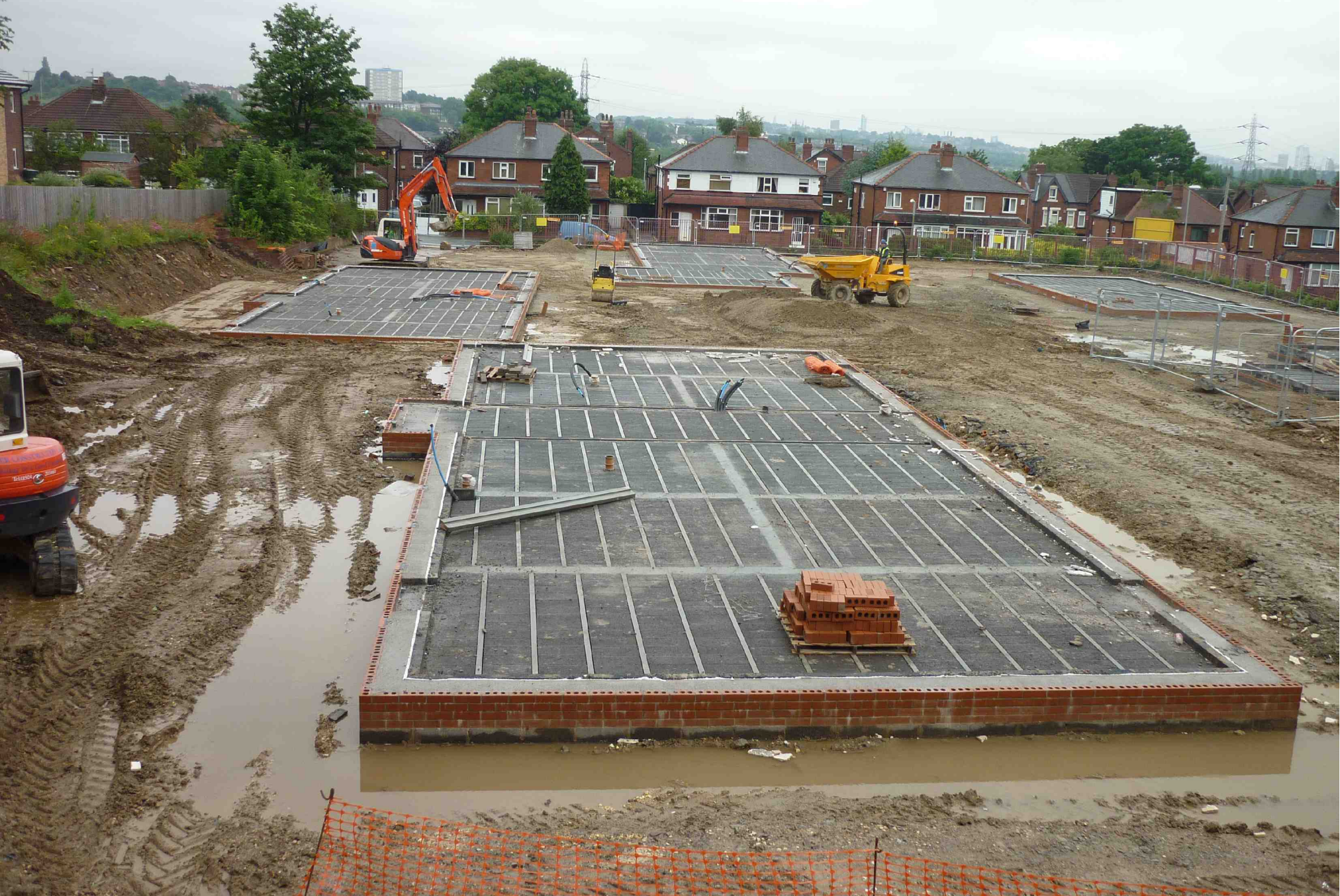
10/07/2012 Foundation & sub-floor complete (for most blocks)
